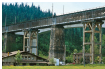
Railway viaduct, Ormaiztegui
